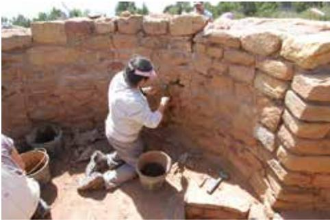
**An Ancestral Lands intern uses the painstaking process of replacing the surface layer of mortar between stones, called “repointing,” to weatherproof precious walls.**
